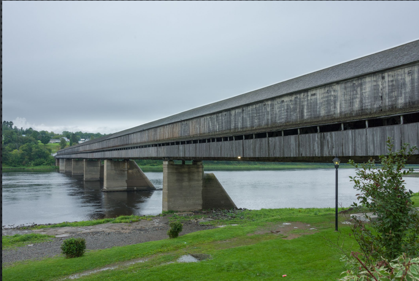
HARTLAND COVERED BRIDGE – NEW BRUNSWICK – 391 M / 1,282 FEET
