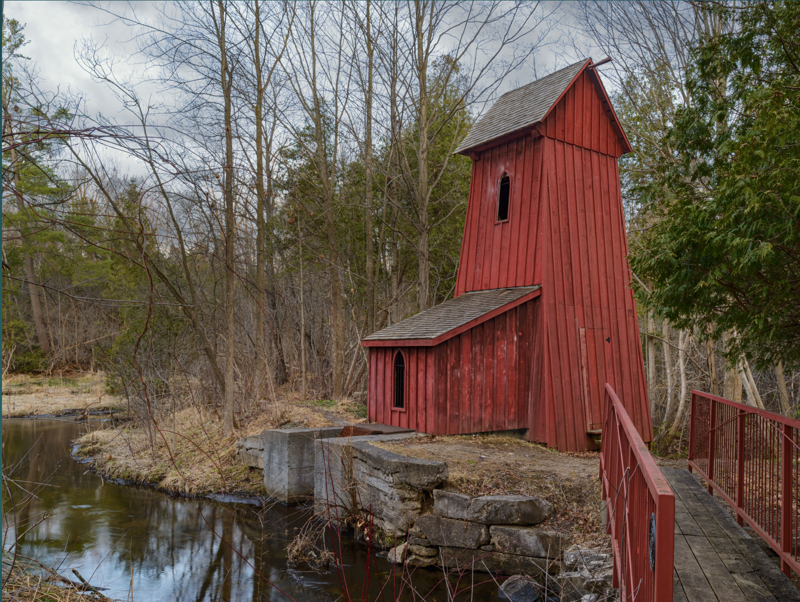
Blair Mill Sheave Tower - Early Spring, Cambridge, Ontario – April 2014
