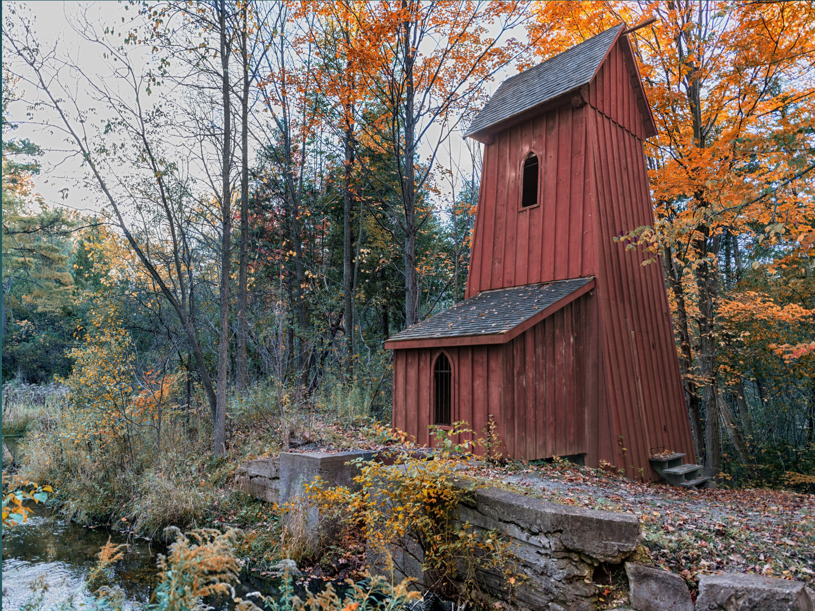
Blair Mill Sheave Tower - Fall, Cambridge, Ontario – October 2013
