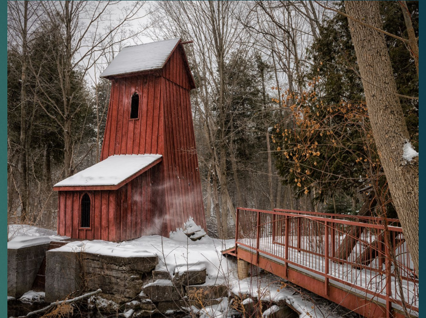
Blair Mill Sheave Tower - Winter, Cambridge, Ontario – January 2014
