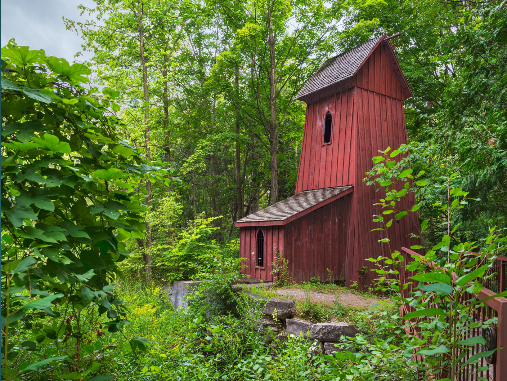
Blair Mill Sheave Tower – Summer, Cambridge, Ontario – August 2014
